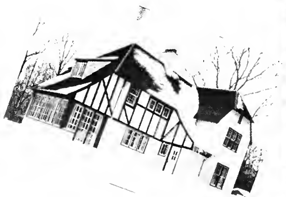
The photograph shows finished results—just two years after planting.
