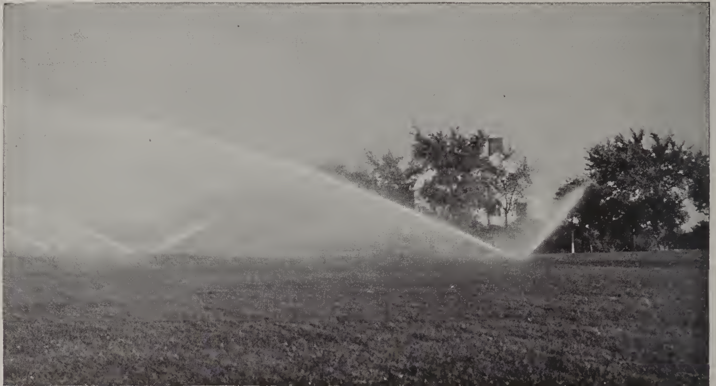
Skinner Fairway System with Broadway Sprinklers in Operation
