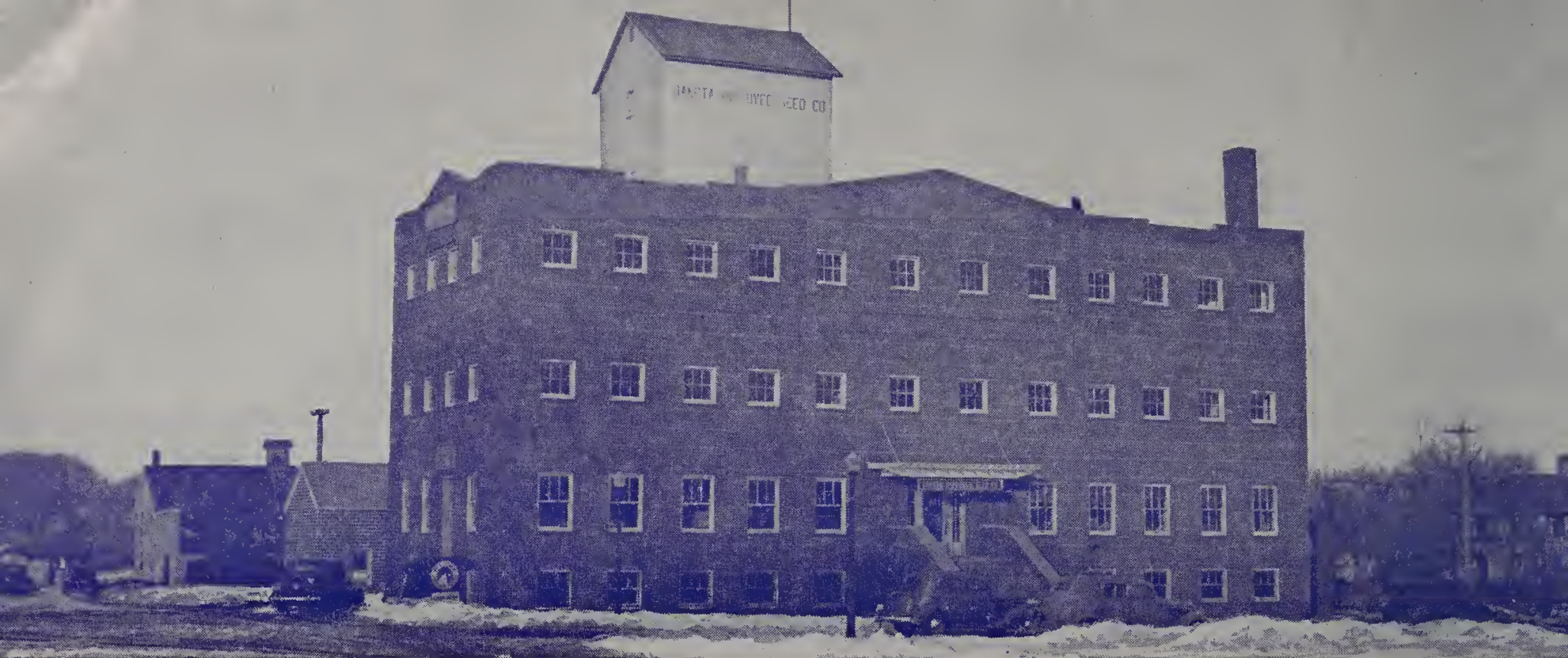
Our Corn Drying Plant and Warehouse, Emmetsburg, Iowa
