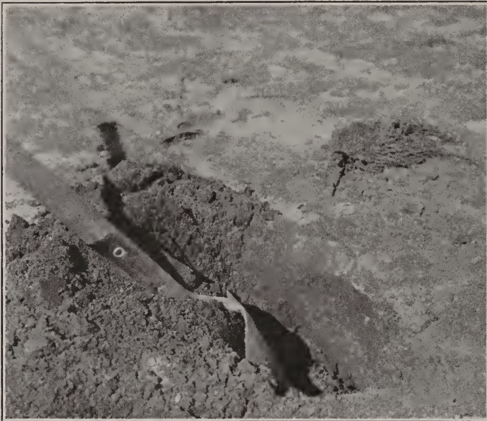
No. 1—First Operation—Making the Hole.
