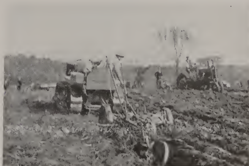
Caterpillar "22" pulling No. 5 Plow with 3-16" bottoms.
