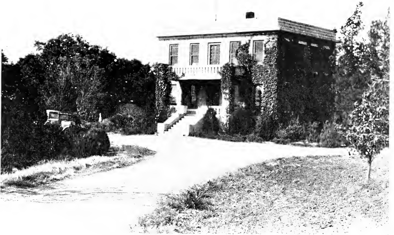
Office Building on Nursery
