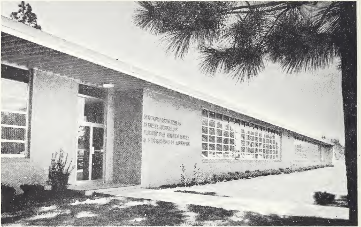
Main entrance and view of front of building (north exposure).
