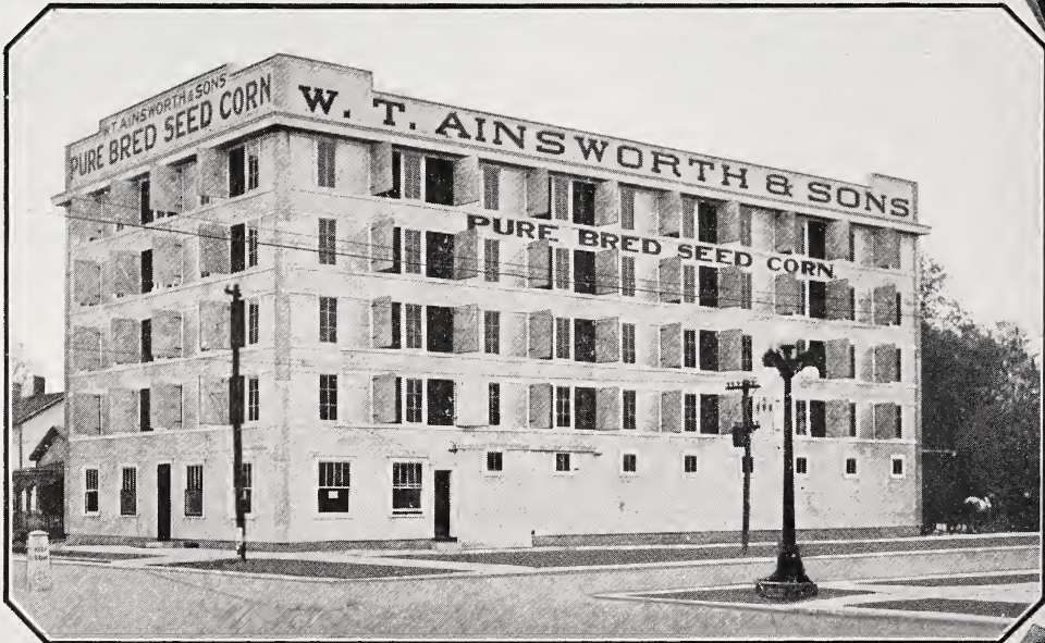
MAIN STREET PLANT SHOWING VENTILATING DOORS OPEN
