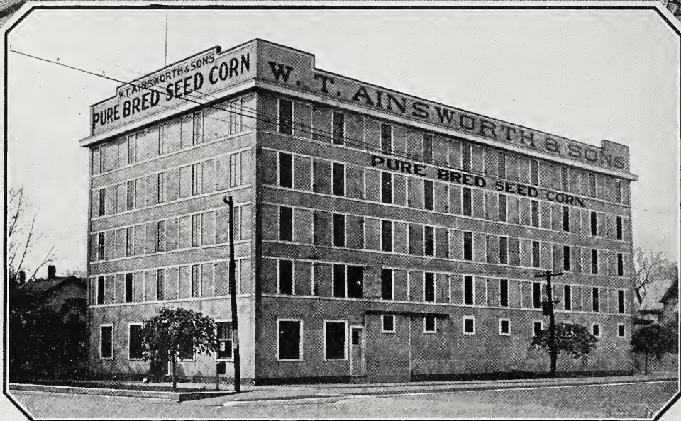
MAIN STREET PLANT SHOWING VENTILATING DOORS CLOSED
