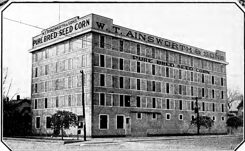
MAIN STREET PLANT SHOWING VENTILATING DOORS CLOSED
