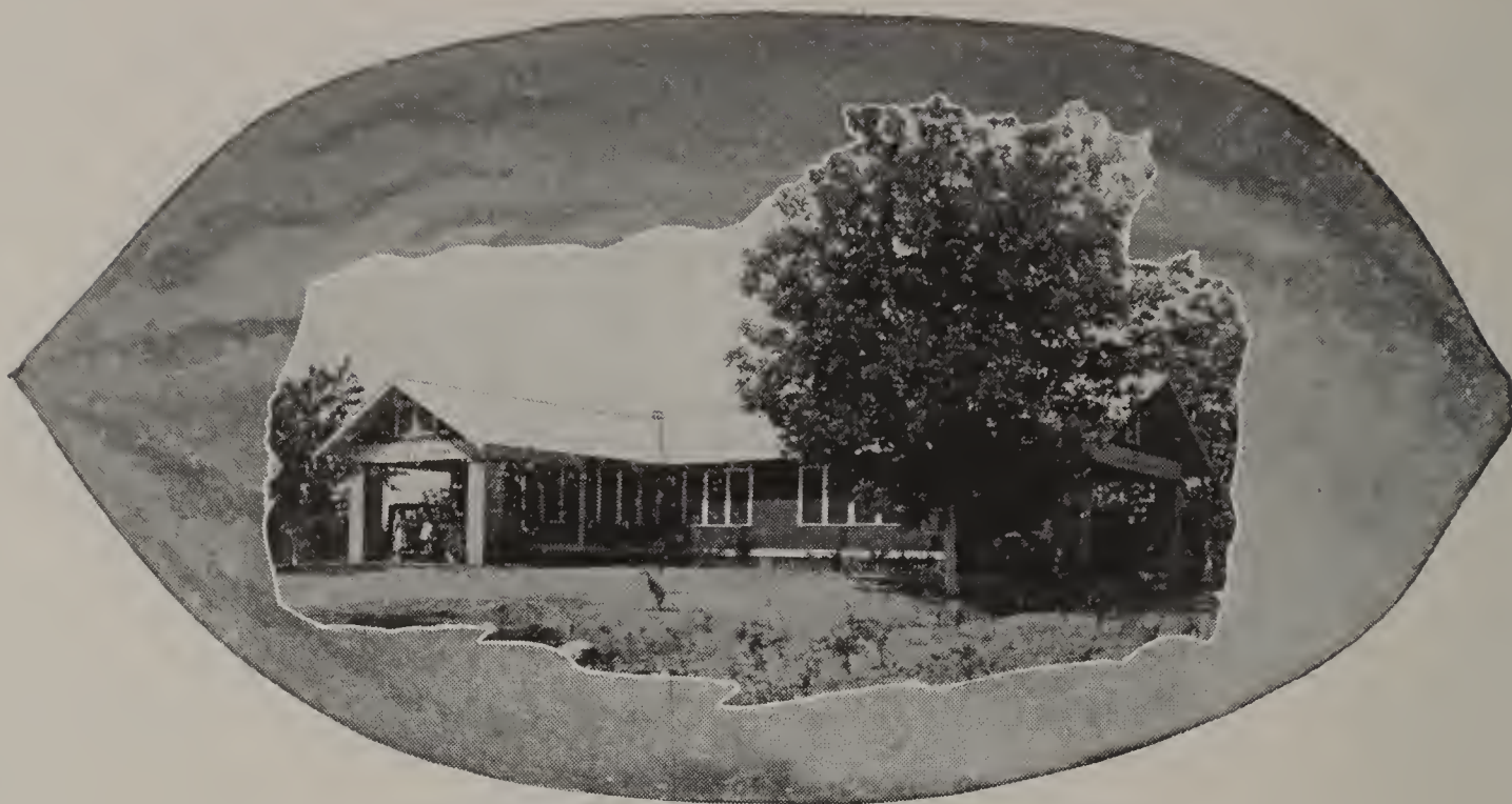
Our Office Building — Notice the Pecan Trees
