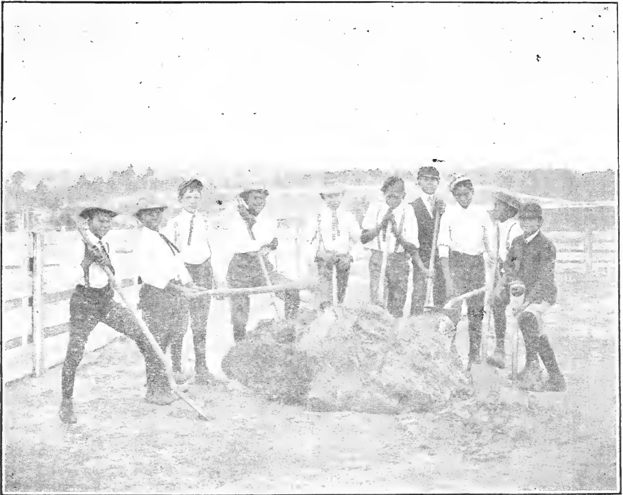
Clearing the Land
