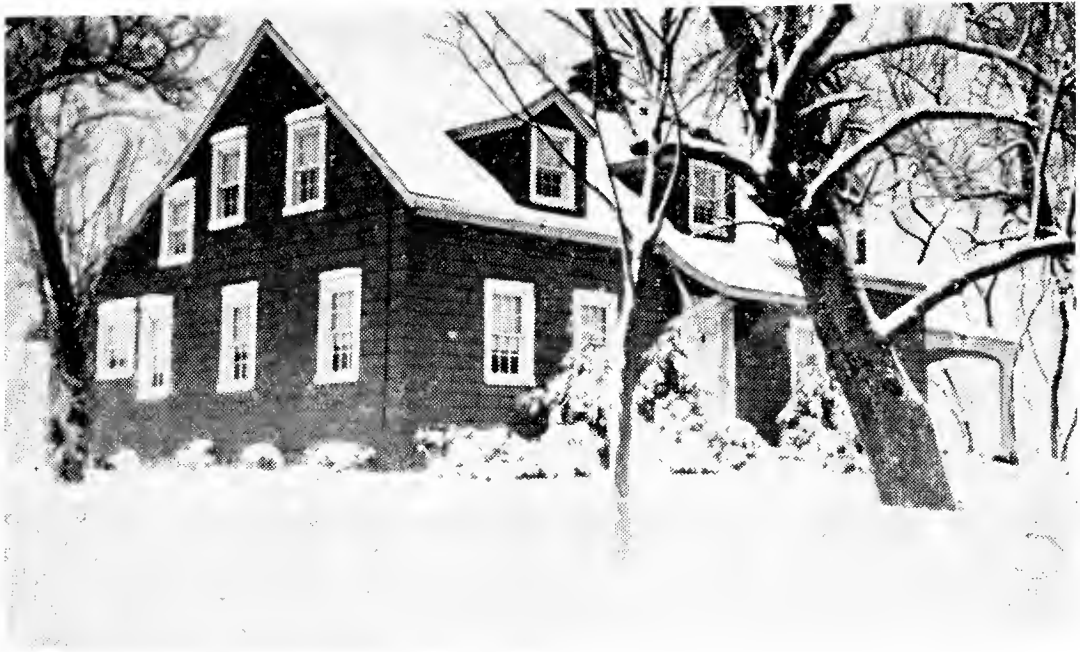
Hurricane Hall in the Winter time
