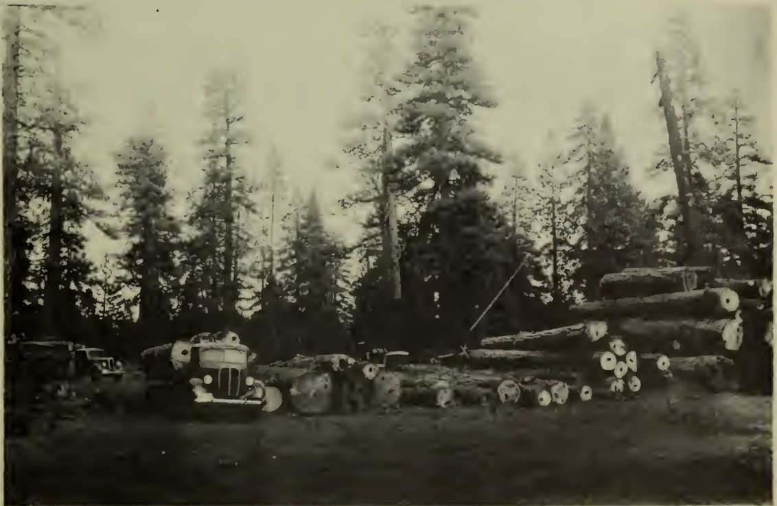
Figure 9. Railroad landing at the Fruit Growers Supply Company's Feather Lake spur. The truck haul is 22 miles.
