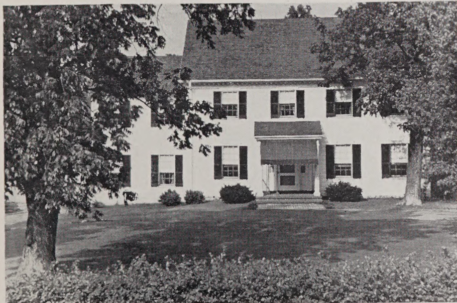
Residence of Dr. and Mrs. Charles Garr, Deepwood
