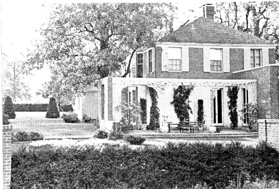
Rear of Residence, Mrs. Christian deWaal, Barrow Road
