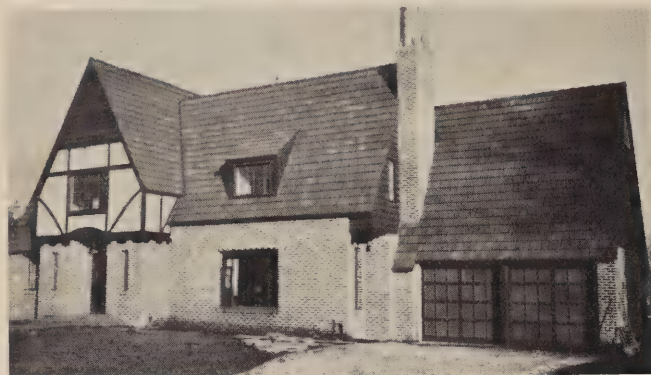
Observe how barren this house looks without Shrubs and Trees and proper landscaping.
