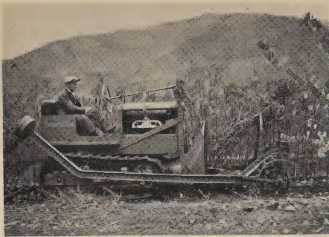
C. & O. CATERPILLAR power tree digger. This modern machine does the work of eight to ten horses. It does a better job and gets all the roots without injury to trees.
