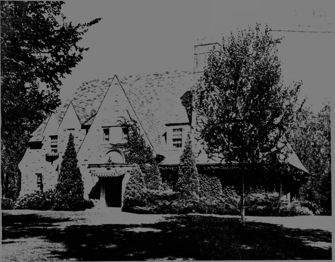
ONE OF OUR WELL PLANTED HOMES.
