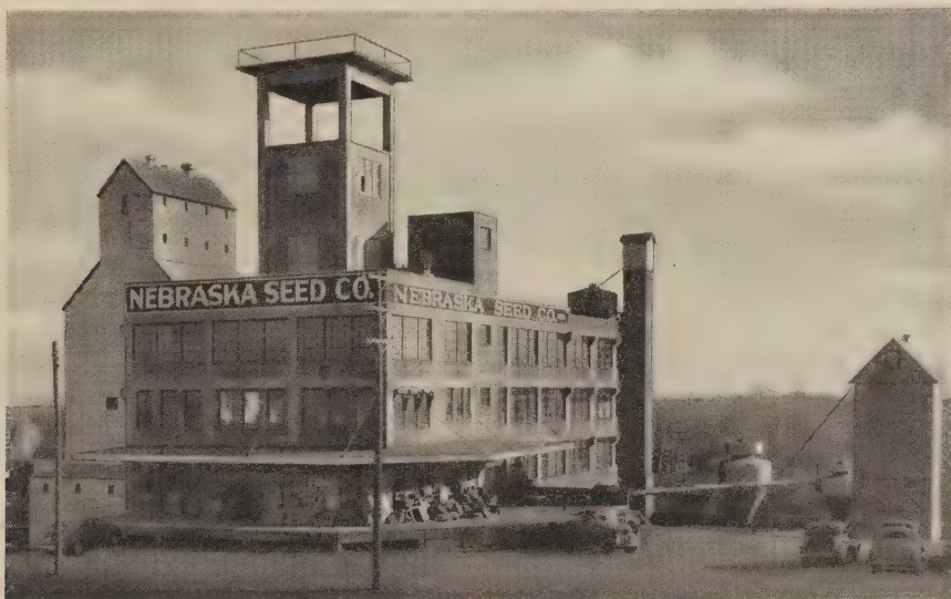
Main Building, Executive Offices, Laboratory and Elevator
