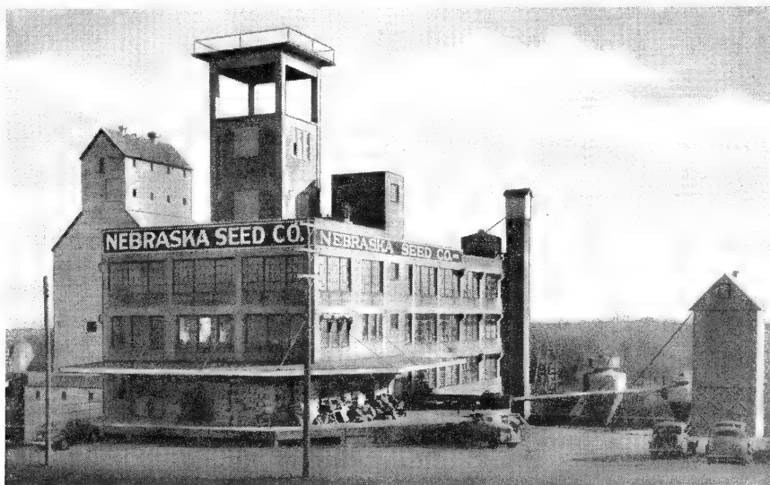
Main Building, Executive Offices, Laboratory and Elevator
