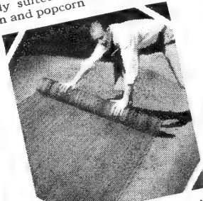
Erosionet —An open-mesh fabric that helps make grass grow even on bald terraces
