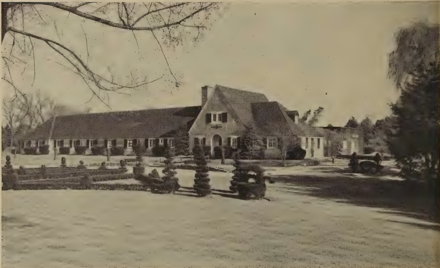
The Wayside Gardens Co. Bulb Warehouse and Office at Glen Head, Long Island, N. Y.
