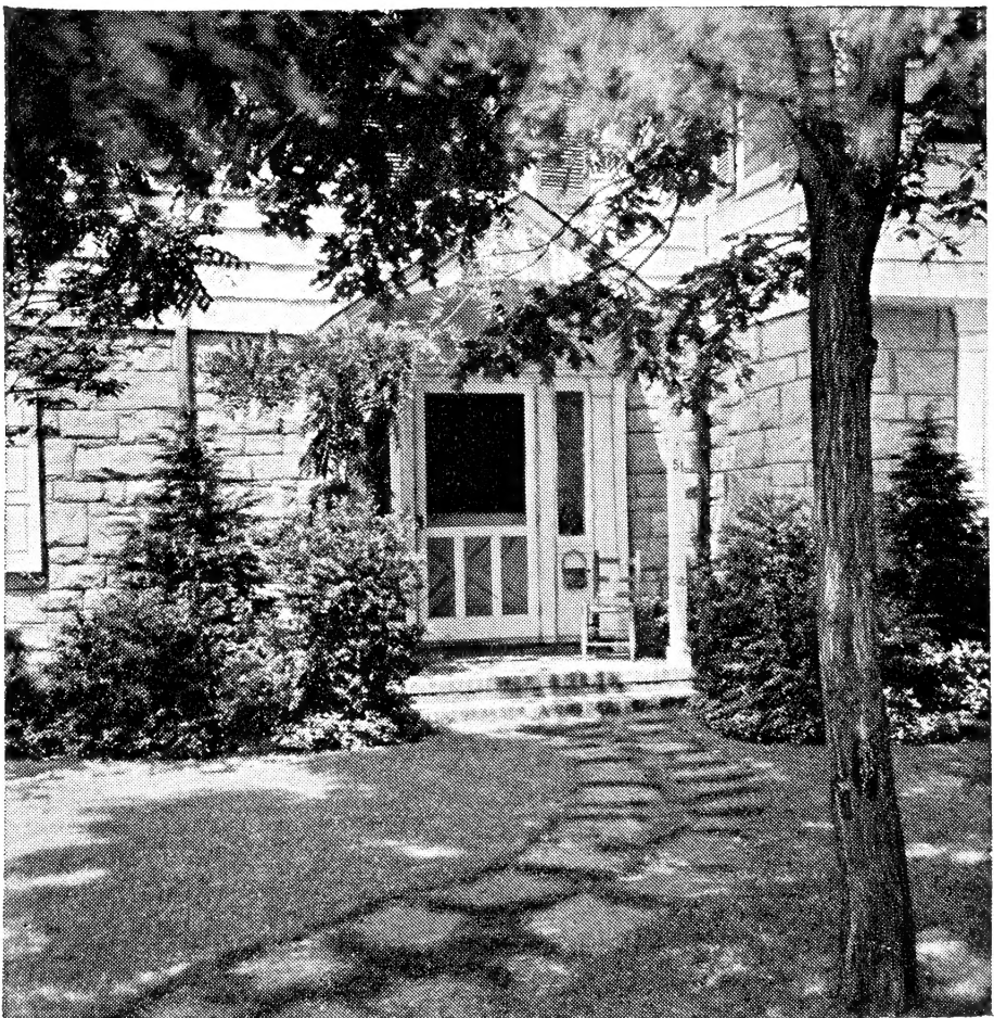
A pleasant home-like entrance approach
