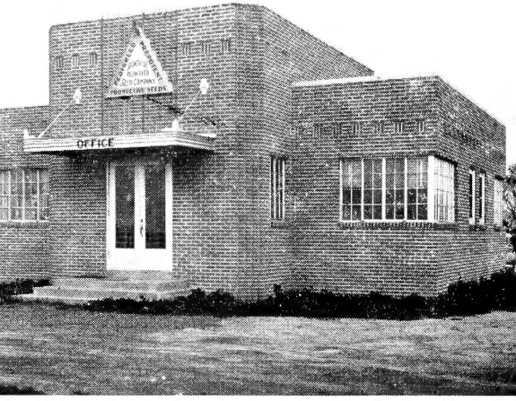
● A familiar landmark at Stoneville Pedigreed Seed Company is its office and administration building, shown above.
