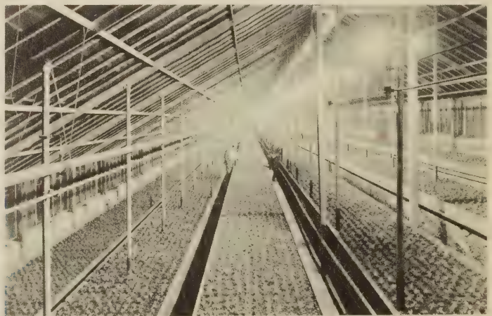
Applying Additional Light to an Entire House
