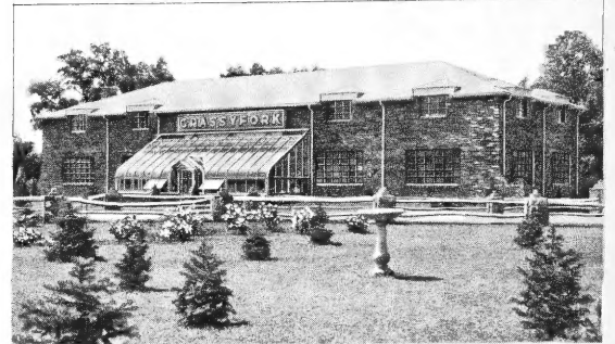
The display building at Martinsville includes conservatories and shows many Grassyfork products.
