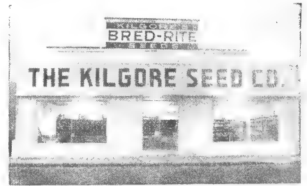
FORT MYERS—1117 Anderson Ave.
