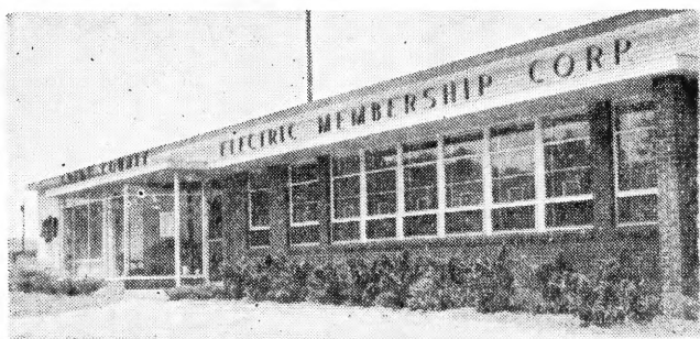
Foundation planting of Suwannee River around an office building.
