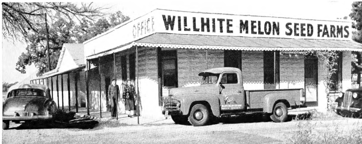
WILLHITE OFFICE AND CLEANING PLANT, POOLVILLE, TEXAS
