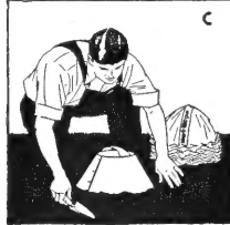
Now cover flange protruding from Hotkap Setter with soil, thoroughly but lightly with your trowel.
