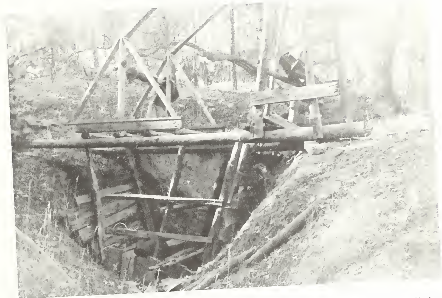
Abandoned mine shaft on Sequoia National Forest, California. Mining regulations will provide for cleaning up mine sites and fencing hazards.
