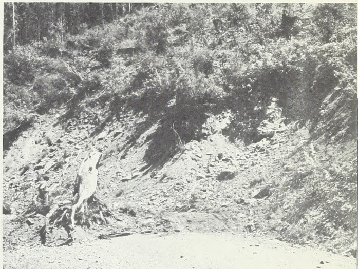
Figure 3.--Backslope failure in an area of soil derived from andesite colluvium.
