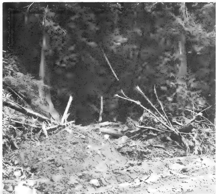
Figure 7.--Debris which blocked the culvert and caused several feet of material to be deposited on the road surface. (Road, in foreground, has been repaired.)
