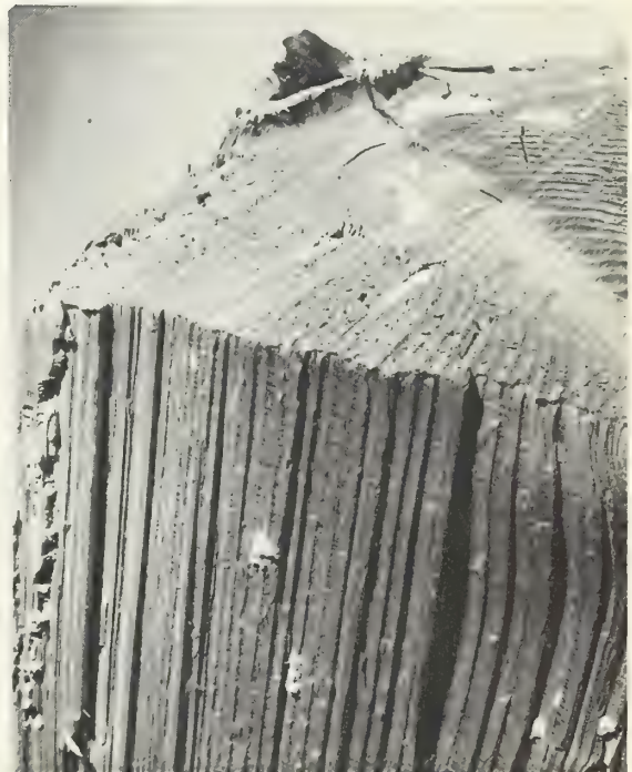
D. Flatheaded borer damage extending to near center of otherwise sound heartwood of tree dead 7 years.
