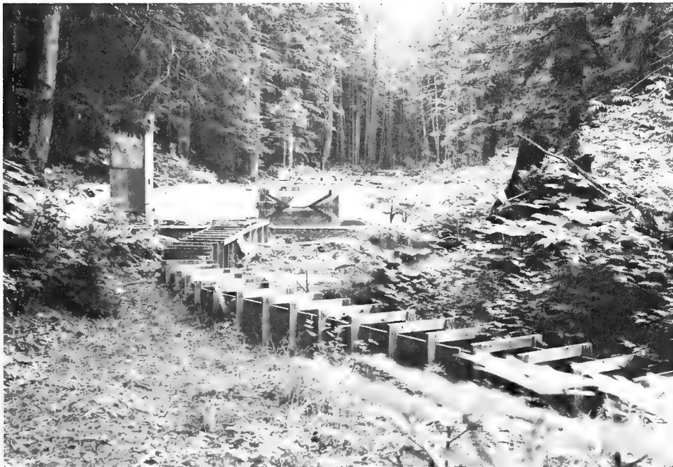
Figure 4.--Intake flume, stilling basin, and outlet to channel showing V-notch weir and gage house.
