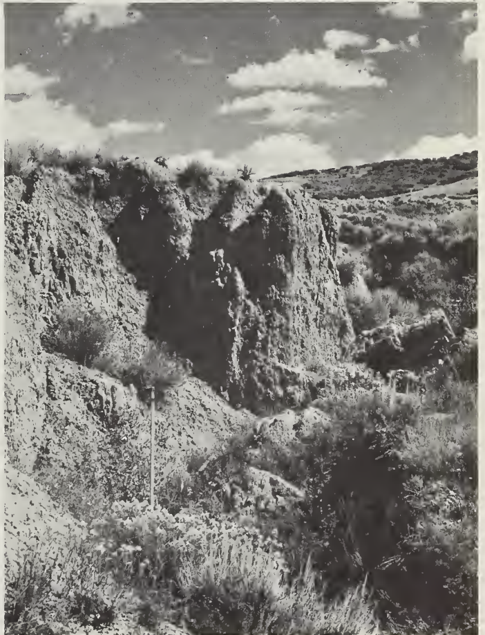
Figure 14.--Piping gully side slopes break off in vertical cleavage lines. The soil masses are dumped on the opposite side slope. These slopes of deposition are invaded by vegetation, while the gully flows are forced toward the piping slopes. The length of the rod is 5.5 feet.
