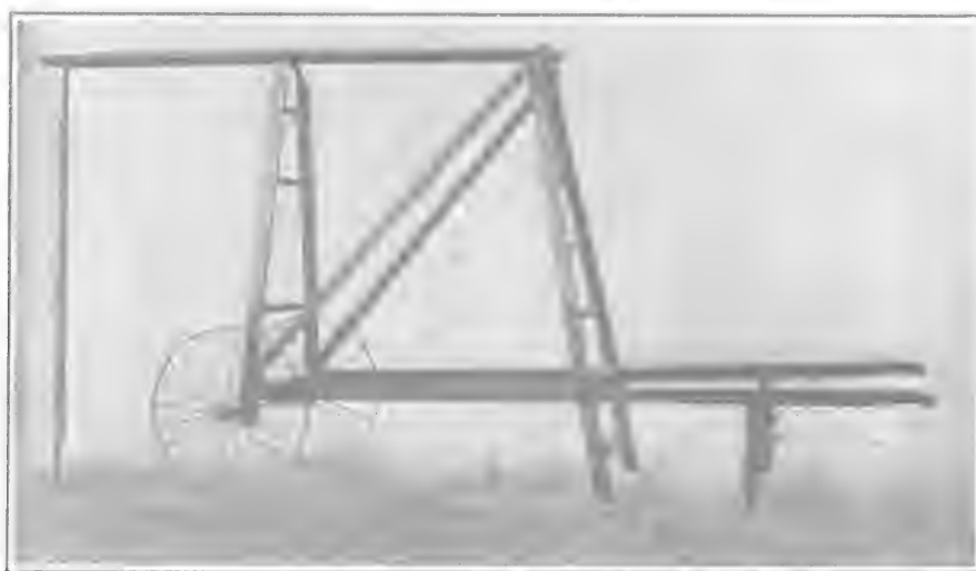
Fig. 6. Portable Orchard Ladder Ready for Use. The running board enables the picker to cover a wider range than would be possible with the ordinary step ladder.
