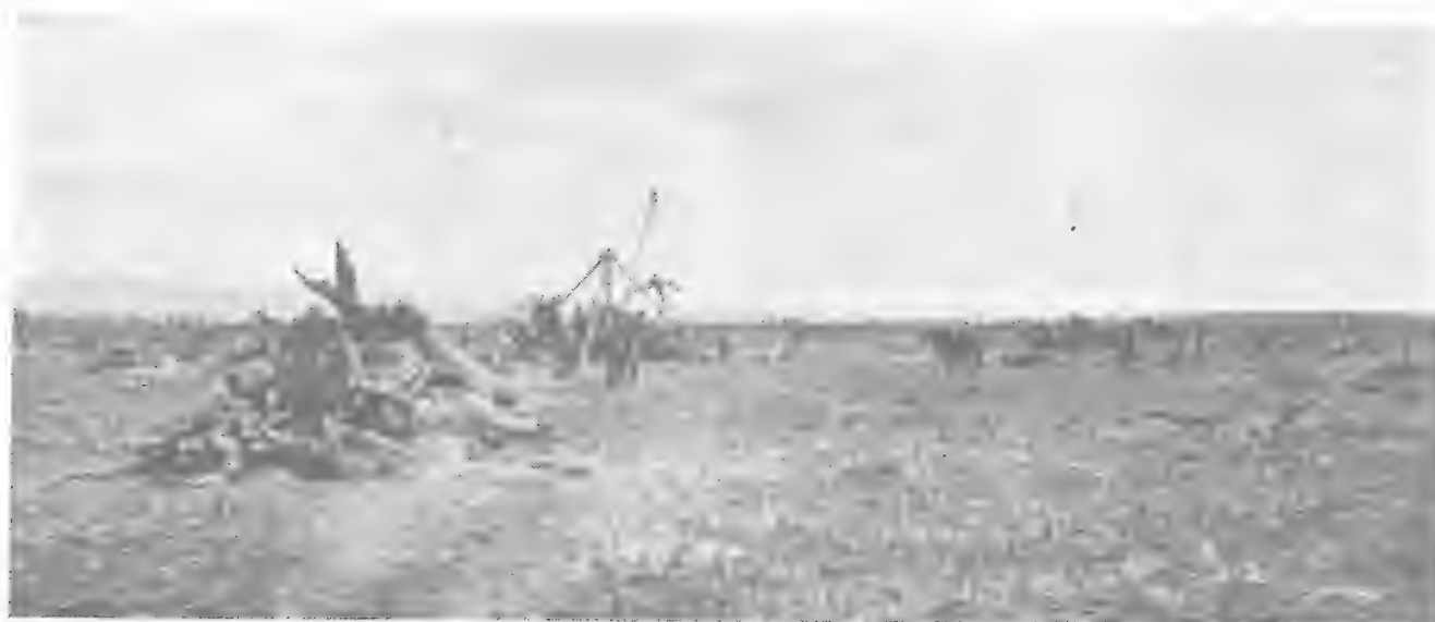
Fig. 1. Piling Stumps with a Derrick before Burning.
