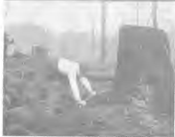
Fig. 3. Beginning the Boring of Holes Under Stump for Blasting.
