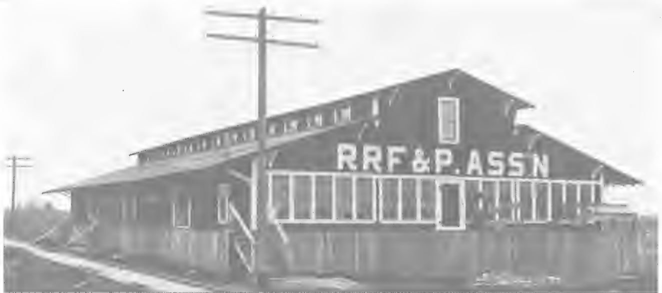
Fig. 10. A Warehouse and Packing House of the Rogue River Fruit and Produce Association, Medford, Ore. Note the excellent provision for light and ventilation.
