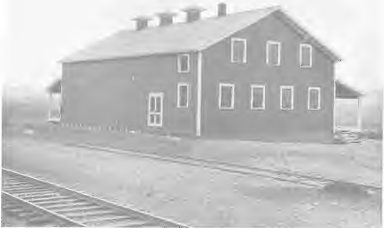
Fig. 9. Combined Storage and Packing House of J. T. Baird, Riverside District, Mabton, Wash. Note galvanized iron ventilators in concrete foundation. This house has a covered platform on two sides.
