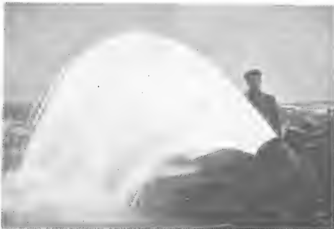
Fig. 5. Artesian Well of Mr. H. R. Lince, Pomona, Washington. This well is 400 feet deep. The pressure is 60 pounds per square inch and delivers 2,250 gallons per minute through an 8-inch pipe. The altitude is 1,250 feet. The well irrigates 500 acres 220 feet above the Yakima River.
