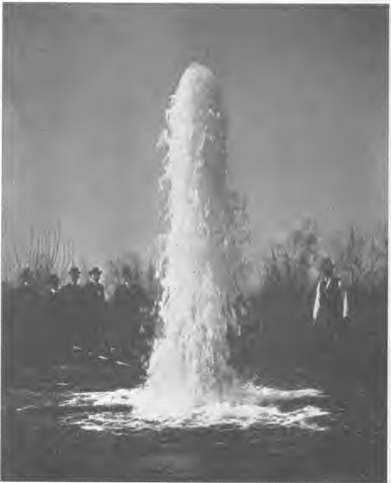
Fig. 3. Artesian Well Near Walla Walla, Washington. 579 feet deep with flow of 2,224 gallons per minute. 62 pounds pressure.
