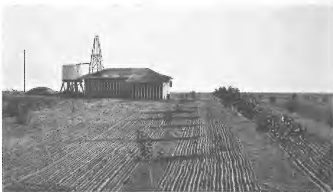
Fig. 4. Pumping Plant of Mr. F. B. Allard. Standpipe to left has a sprinkler at the top.
