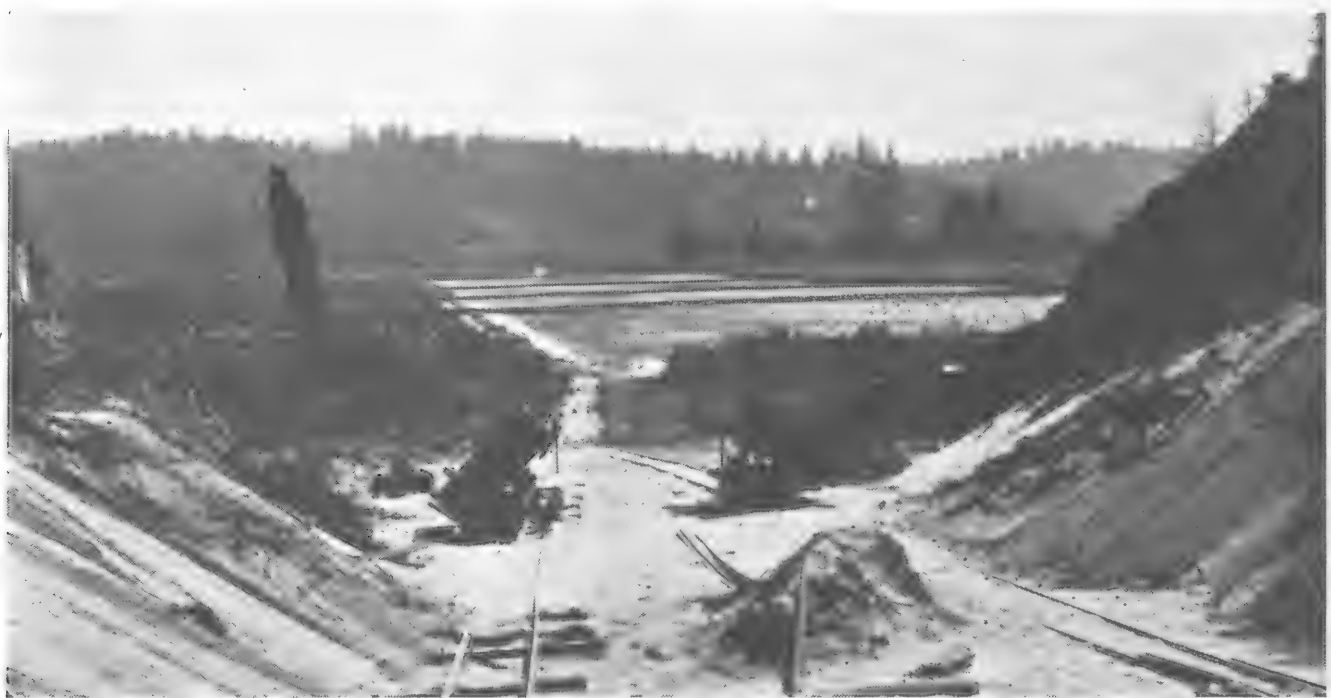
Fig. 1. Part of a Thirty-Acre Tract of O. B. Estes of Astoria, Oregon. In the foreground is the sand pit from which the bog was sanded and also the track and cars used in sanding. A large lake of about 300 acres is at the far end of the bog and is about six feet below the bog. It is intended to water from this lake for irrigation and flooding and to drain all the water back into the lake.
