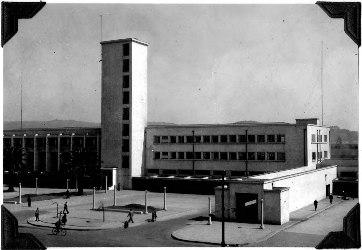
New railroad station, Concepción.
