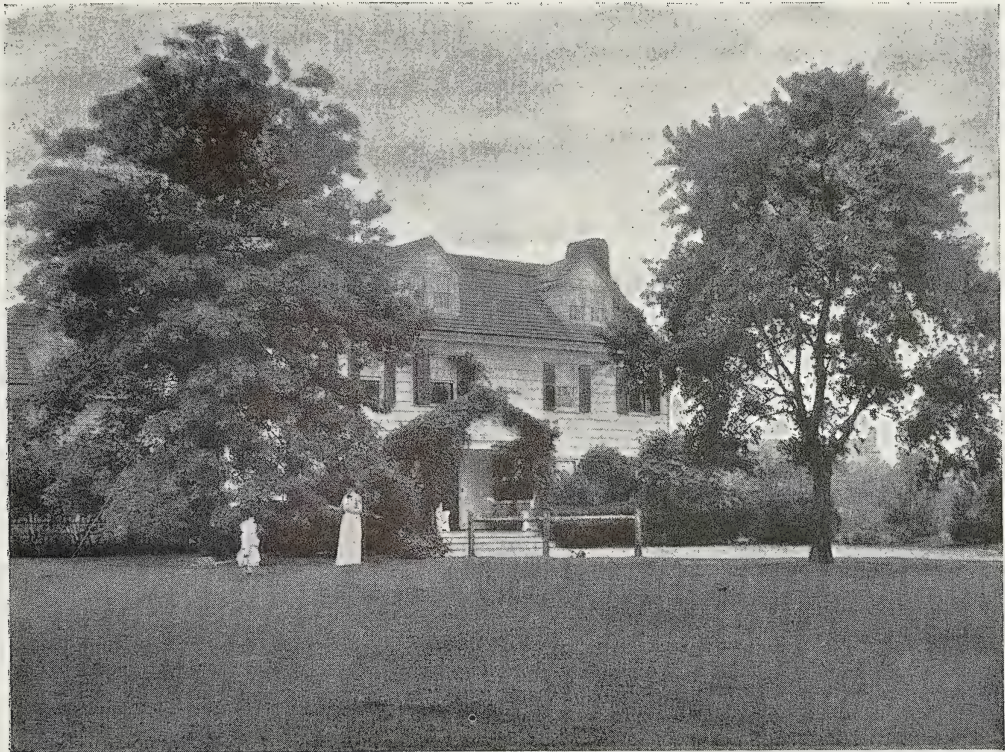
Residence of Mr. John L. Lawrence, Lawrence, L. I. This new seaside lawn, planted with low-spreading Pin Oak, Wild Cherry, and old Dwarf Boxwood, has immediately the charm and repose of a half century's growth. Photographed four years after planting.
