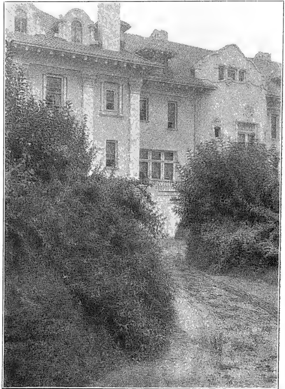
A new solution of the service court and laundry paddock problem. Court sunk to the basement level and having vertical walls of foliage, thus preventing a view from the street. The walls are built at a steep angle by laying sod, like bricks, with Honeysuckle between, and weeping Forsythia at the top. Residence of Mr. Alexander C. Humphreys, North Country Colony, Glen Cove, L. I.
