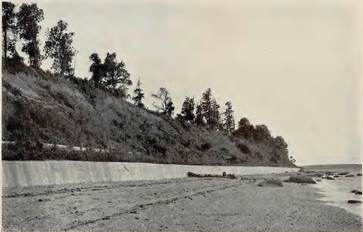
Bluff at Red Spring, Glen Cove. In the winter the loss of land at the top is rapid, but can be prevented by close planting with small evergreens (as described under Pitch Pine), mixed with various deciduous shrubs and vines. Partial death of the trees at the top could have been checked by low planting about their roots. Concrete sea-wall and jetties of boulders.
