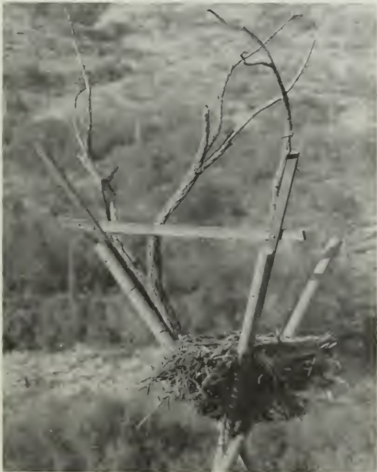
Figure 3.—Superstructure of the nesting tripod showing apex joint, 2 by 4 framework, perch branches, and nest materials.
