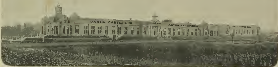
Carters Head Offices, Warehouses, Laboratories, and Testing Grounds, Raynes Park, London, England.
