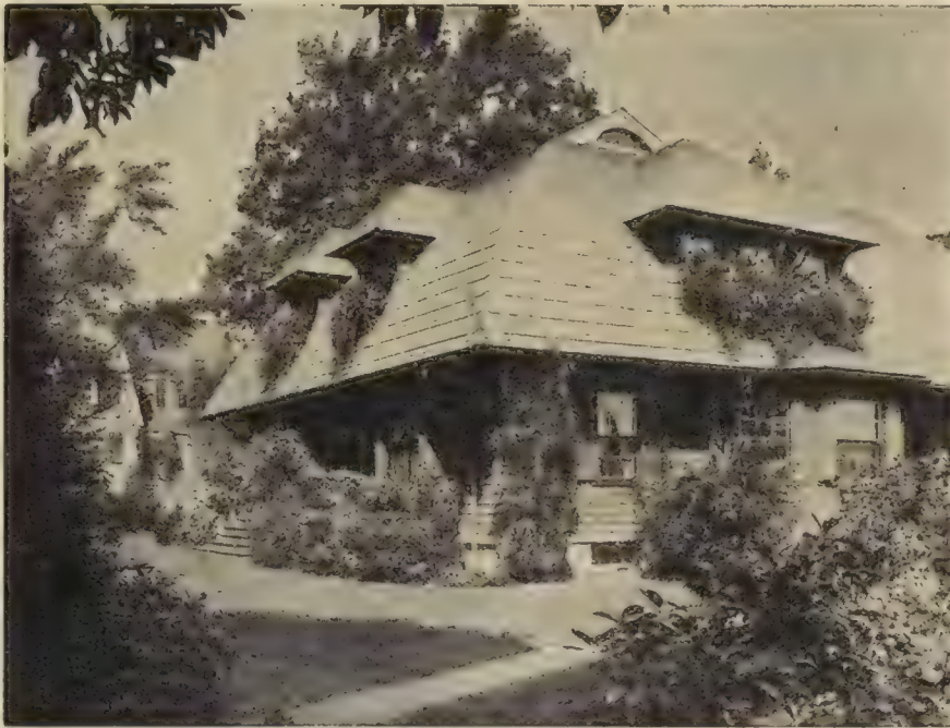
EFFECTIVE TREATMENT OF A BUNGALOW
