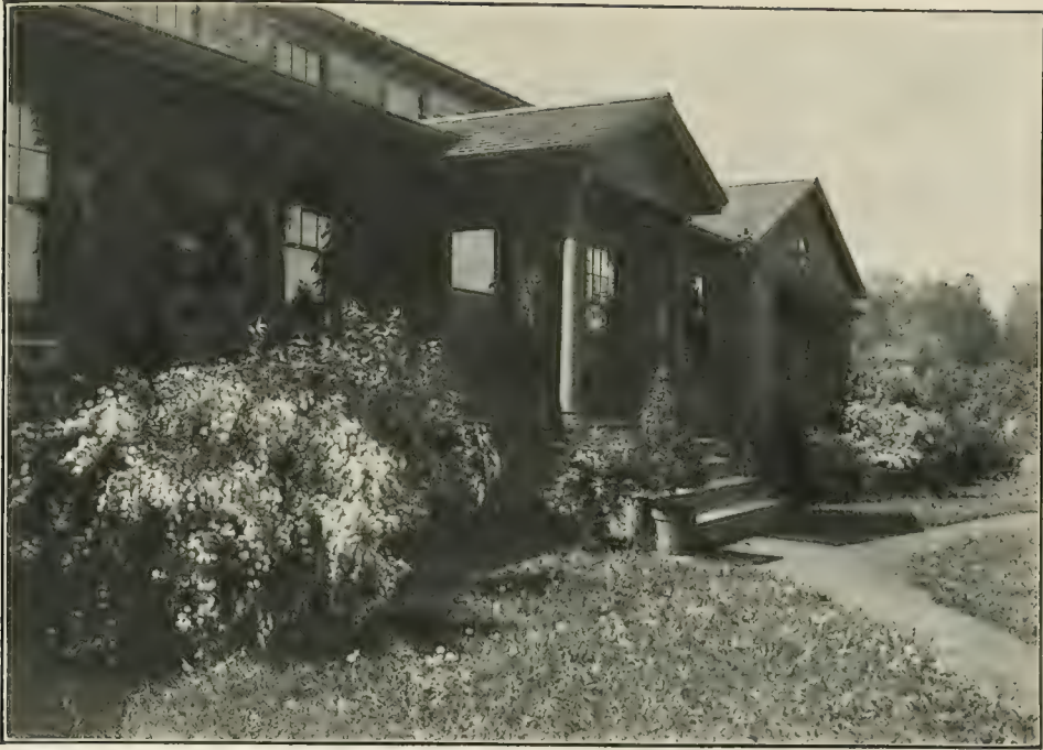
Arrangement of Shrubs in front of our office buildings
