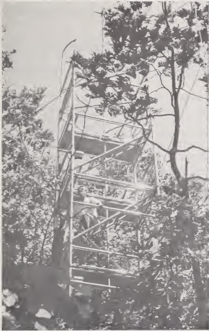
Figure 4. Instrument tower with aspirated thermistors and psychrometers.
