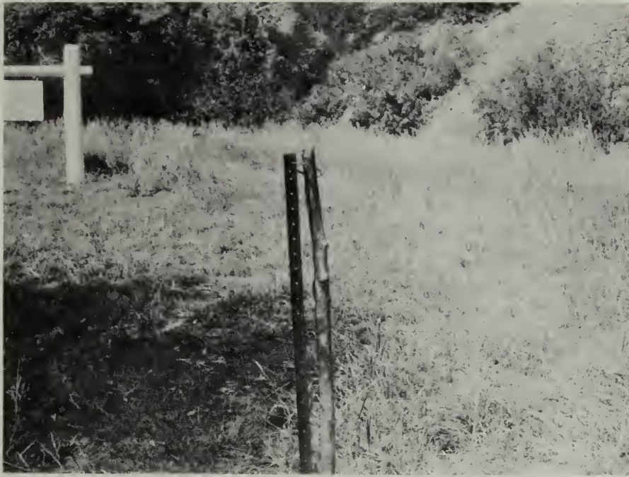
STAY HELD IN PLACE WITH A LOOP WIRE THROUGH HOLE IN METAL POST
