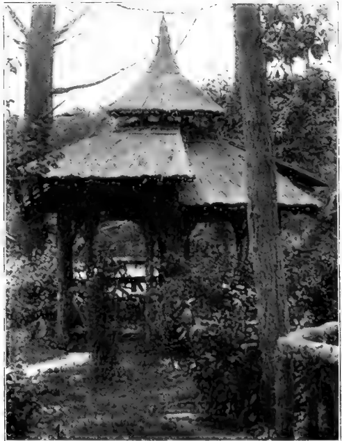
SUMMER HOUSE, THATCHED STRAW ROOF
