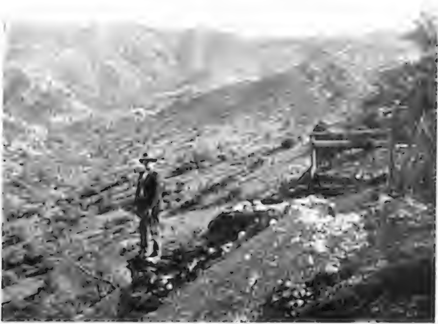
Fig. 1 No. 6 Workings and Radium Ridge forming the sky-line
