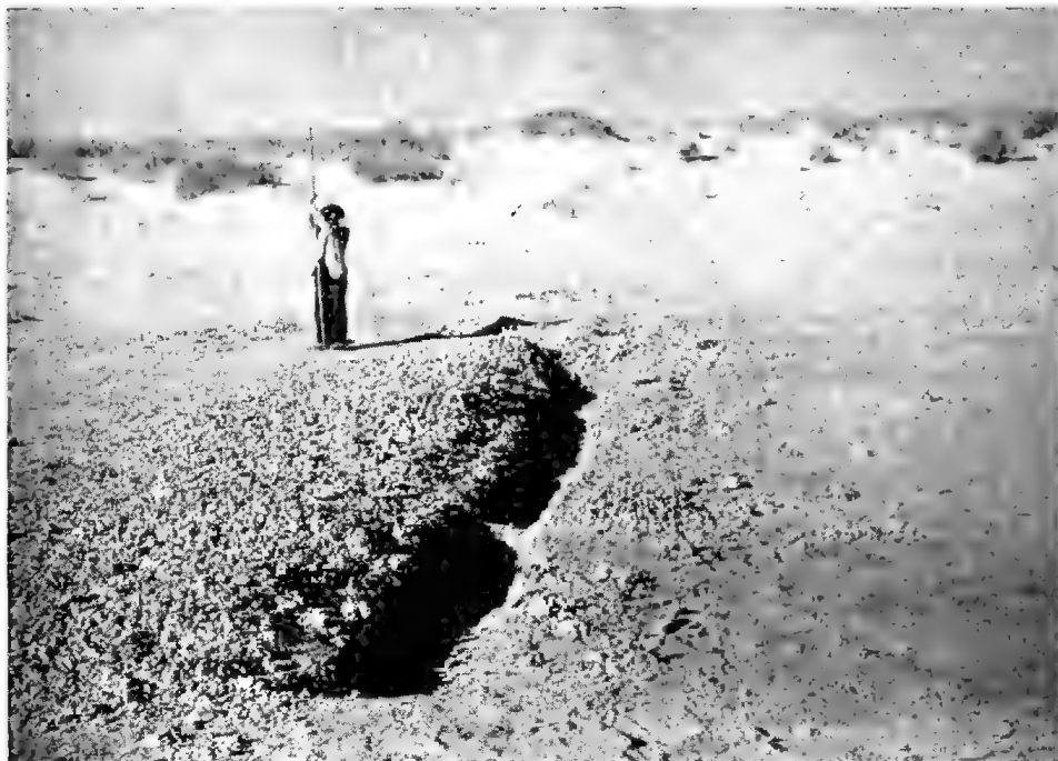
Fig. 1.—The costean at Location W, showing (left) the rod being withdrawn from the bore.
