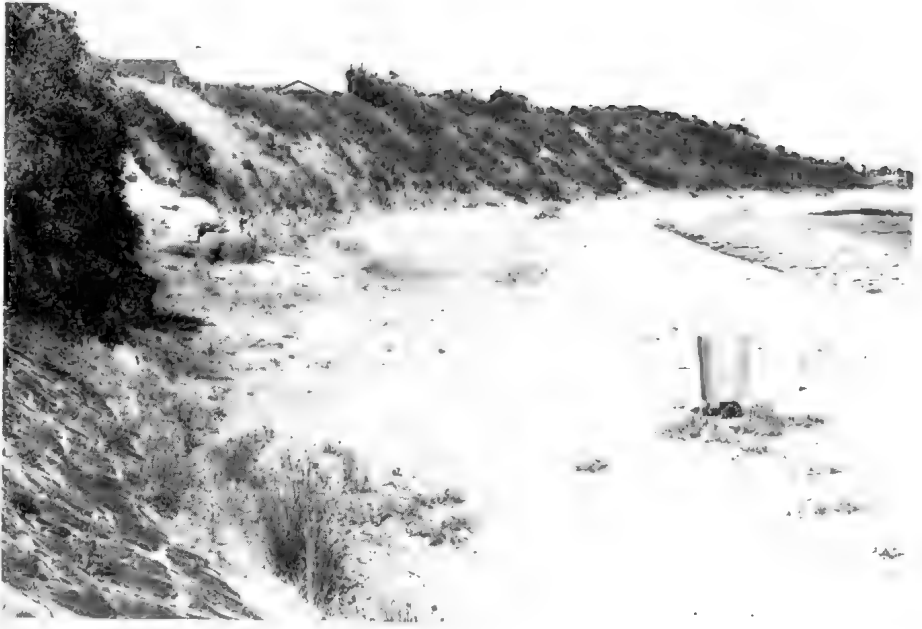
Fig. 9. The bluffs south of Quiet Corner, Black Rock, were being undercut until an artificial beach was emplaced to protect them from erosion in 1984.
