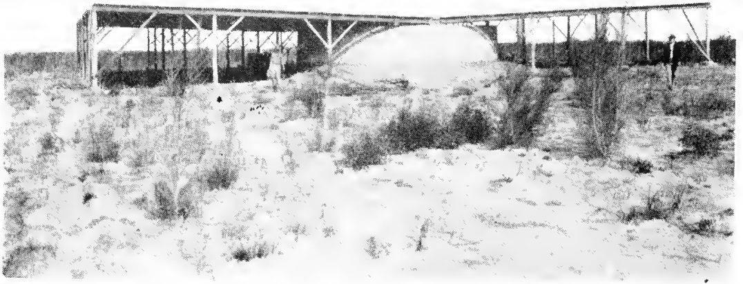
Fig. 6.—A roof catchment, about 40 miles west of Kumarl on track to Mt. Holland. (Photo. by Prof. J. A. Prescott.)
